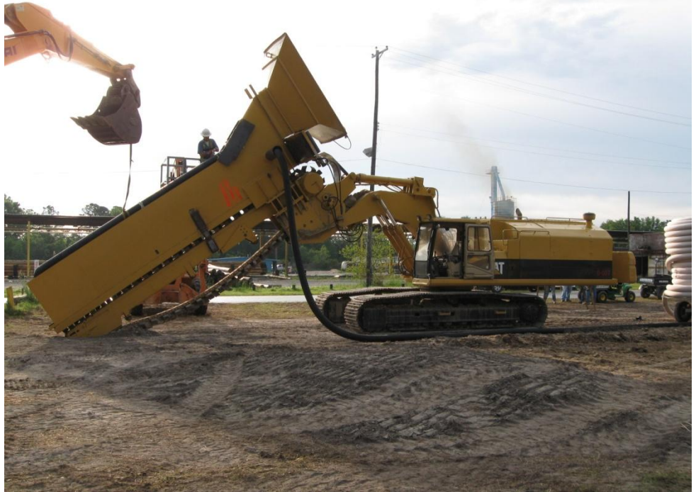
HSSI prepares a LINEAR CONTAMINANT REMEDIATION SYSTEM (LCRS) for installation. Shown is the vertical riser, the sand backfill chute, the Horizontal Well and the delivery mechanism. This installation was located at an EPA Superfund site.
