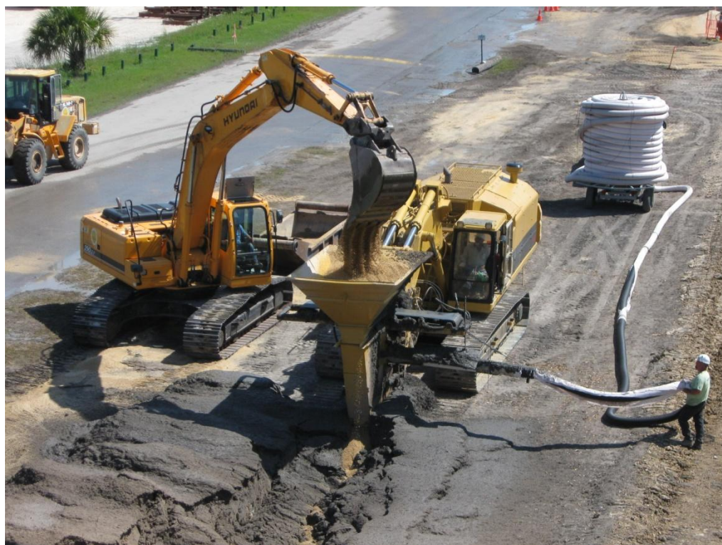
Overhead view of LCRS being installed with filter media. The one pass process excavates, lays the recovery pipe and backfills.
