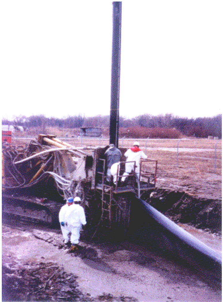
Installation of Polywall Barrier System at EPA Superfund site was 30 feet in depth and one mile in length. Picture depicts loading of a new Polywall segment.
